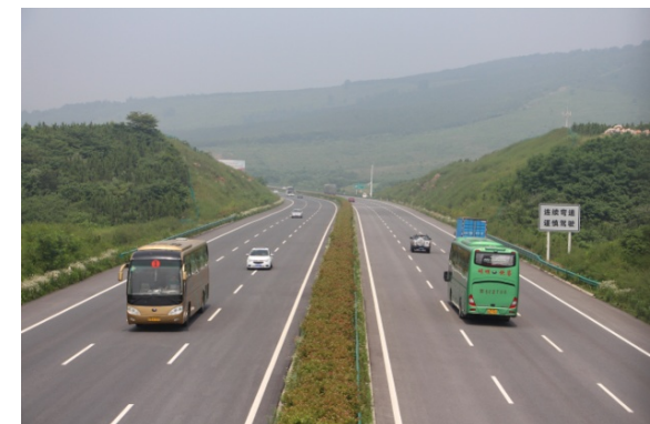
Machao Expressway in Anhui
