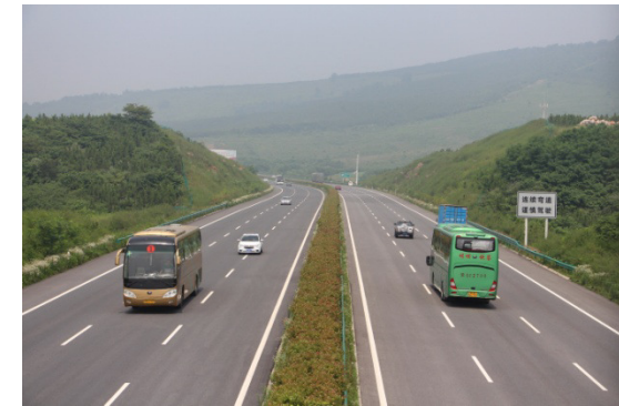
Machao Expressway in Anhui
